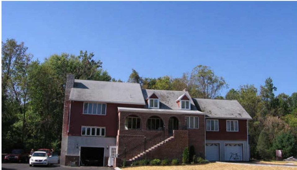
Structure after mitigation. The house has been elevated to raise it above the BFE.
