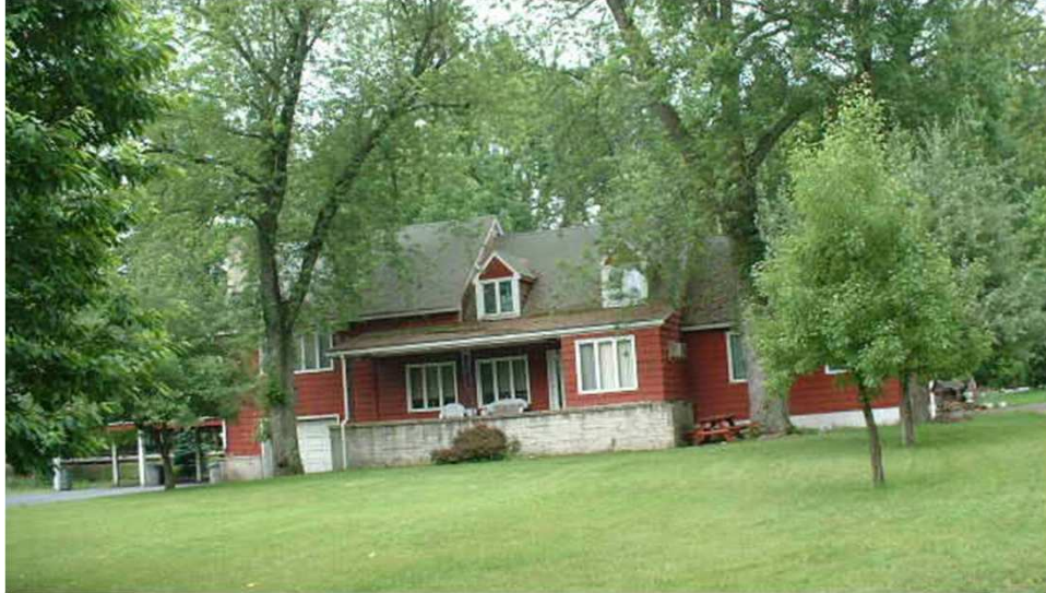
Structure prior to mitigation.
