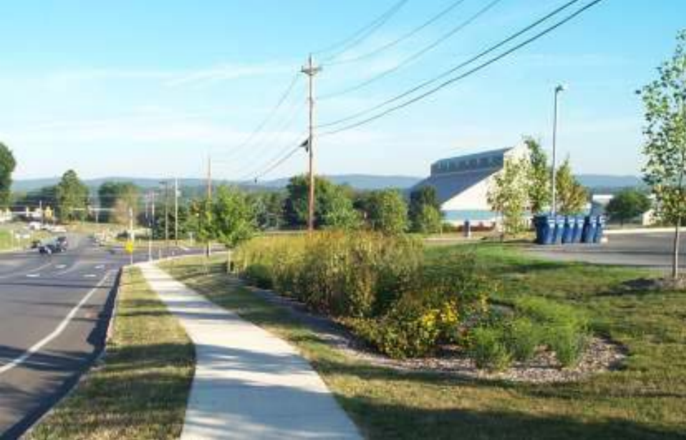
Penn State University Park Porous Concrete Sidewalks
