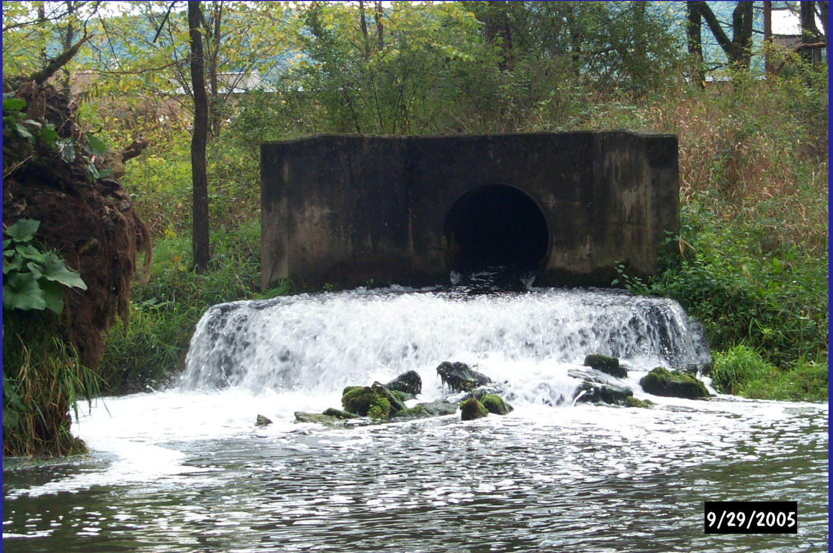
UAJA sewage treatment plant outflow
